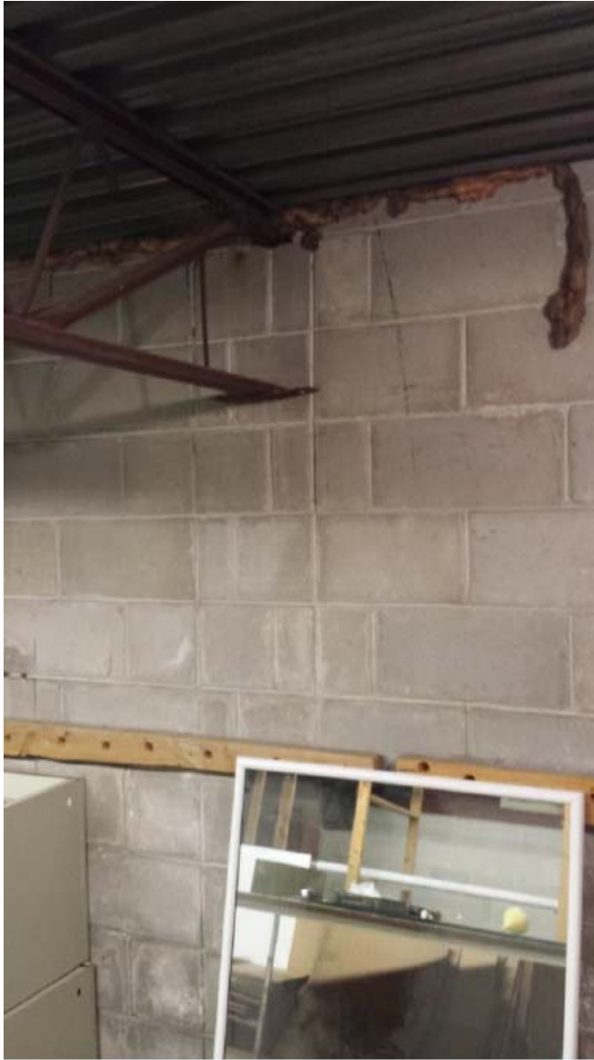
Photo No. 1: OWSJ bearing on south masonry wall.
