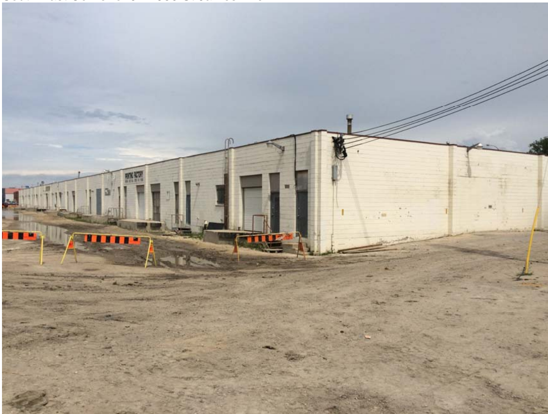
Southwest Corner of 914-950 St James Ave
